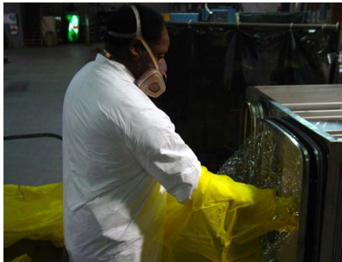
Figure 1-14-note bag is resting on a parallel flat surface and not the floor
